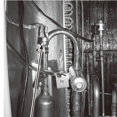
High pressure switch (63H)
